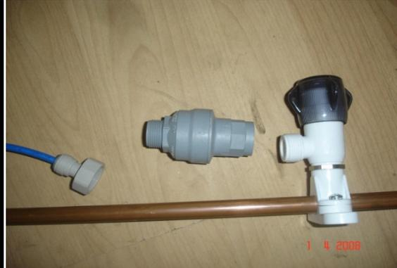
Turn the tap off (If its already off that could be your problem) unscrew by hand the grey cylindrical connector from both ends (tap and pipe) Fig 6.
